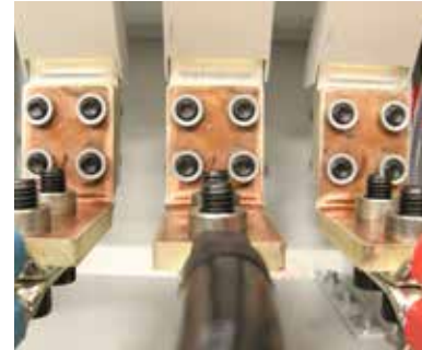
Silver-Plated Customer Connections
